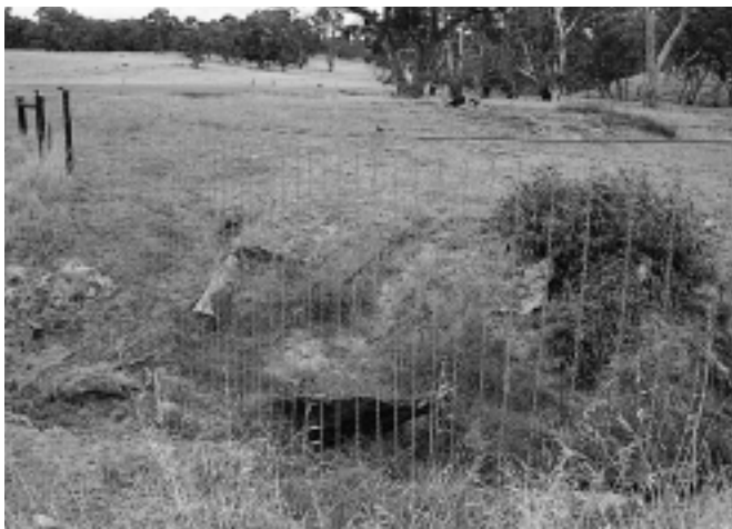
Figure 11: Electrified flood gate.
